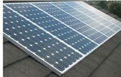
To offset 60,510.06kg/year of CO<sub>2</sub> the installed PV arrays must generate 116,589.72kWh/year of electricity. SAP Appendix M estimates that this can be achieved through the installation of PV arrays totalling 142kWp. This is the equivalent of 568 no. 250Wp PV panels orientated in a south easterly to westerly direction. Note however the MCS method of calculation will give a lower kWp figure for the same level of generation.
